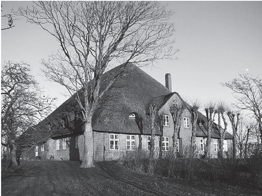
Fig. 8. The Haubarg Blumenhof in the western part of the Eiderstedt peninsula was built in 1790. The supporting construction of the “gulfhouse” consists of six wooden pillars (pinewood). The photograph shows the integrated part of living space, which is oriented to the south. The domestic part with the storeroom for the crop in the centre of the house, in the so called Vierkant between the wooden pillars, the threshing floor and the cowbarn points to the north. Photo: Gerd Kühnast, Interessengemeinschaft Baupflege Nordfriesland & Dithmarschen
